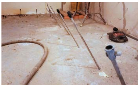
Soil stabilization
